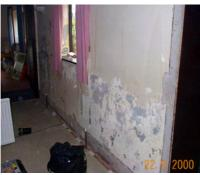
Internal finishes were lime washed which allowed surfaces to breathe and, although it would discolour when damp, it would not peal off the wall like wall paper nor blister like modern paint.
